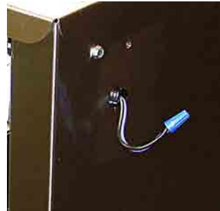
Figure 7: Control connection wires.
