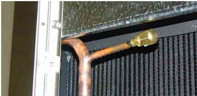
Figure 11: Low side service port.
