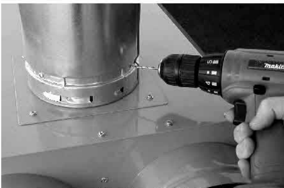
Drill two 1/8-inch holes in the flue
