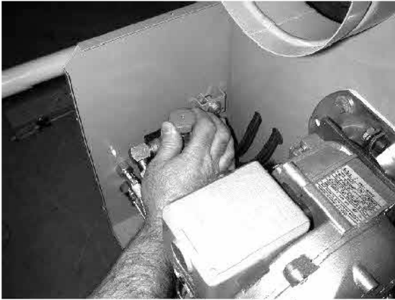
Close the fuel line shut-off valve
