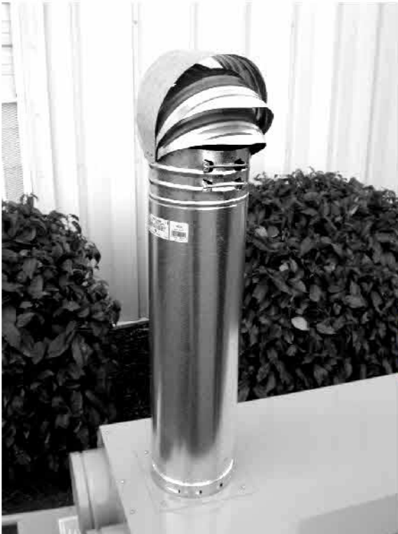
Attach the flue to the Dragon
