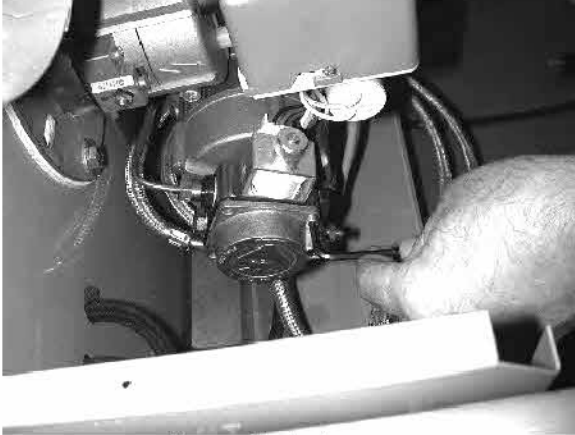
Remove the fuel pump cover
