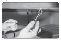
**Step 8:** Pull down on the ratchet rope, lifting the unit in place. We recommend pulling down on each individual ratchet rope 6-12 inches at a time until level.
