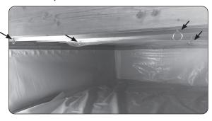
**Step 6:** Position the unit directly below the eye bolts. Attach the four ratchet straps to the pre-drilled holes on the hang kit brackets using the non-ratchet clip end.
