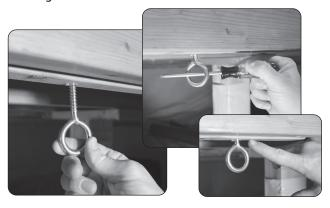
**Step 4:** Distance the second eye bolt 55" away from the first eye bolt on the same joist and screw into place.
