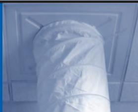
**Ceiling discharge kit** allows condenser-air to be vented to the plenum area above a suspended ceiling.
